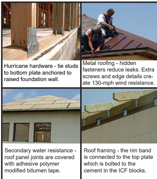
Hurricane hardware - tie studs to bottom plate anchored to raised foundation wall.
